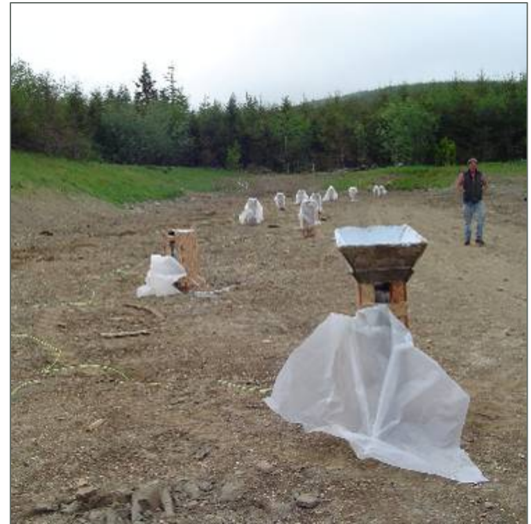
Hoppers for pouring explosives into charge gap
