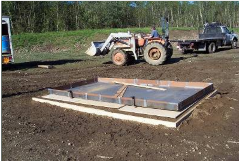
Final shot readied for detonation
