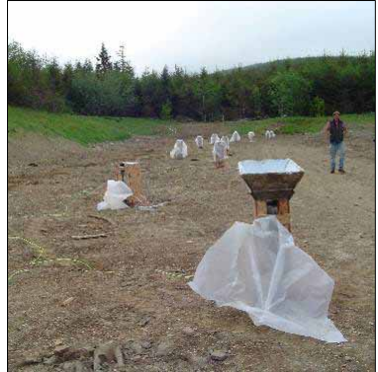
Hoppers for pouring explosives into charge gap
